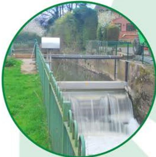
The tilting weir is driven from one side, meaning that the structure didn't need any form of access gantry across the river, with the build-height being half that of the original sluice.
