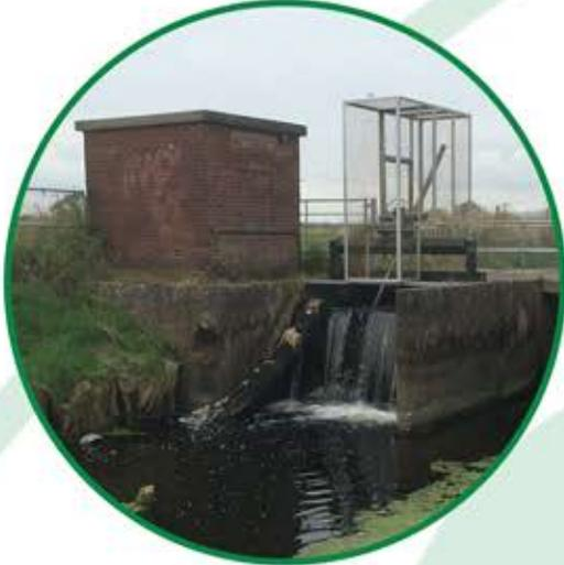
The sluice at Broadway Reen in Newport originally incorporated an open channel and a Tilting Weir, and was identified in 2016 for refurbishment to improve flow control.
