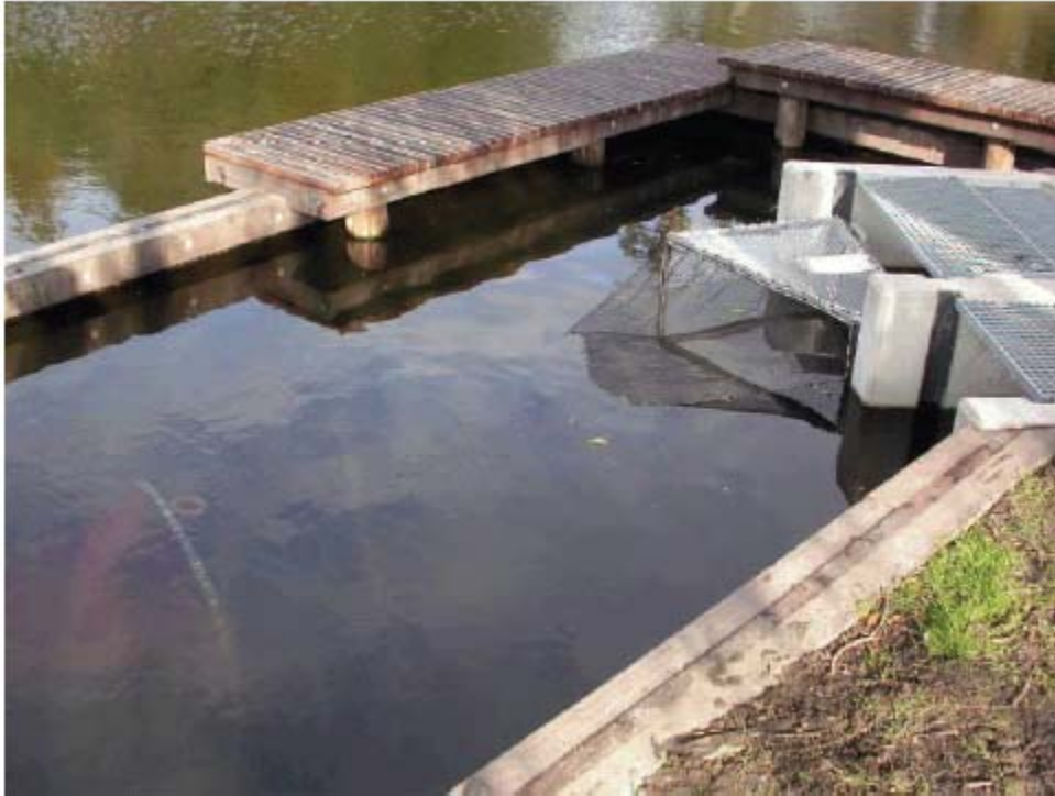
Figure 9 Trapping structure behind the outflow orifice of the Kralingse Plas pumping station (photo: Koeman and Bijkerk).
