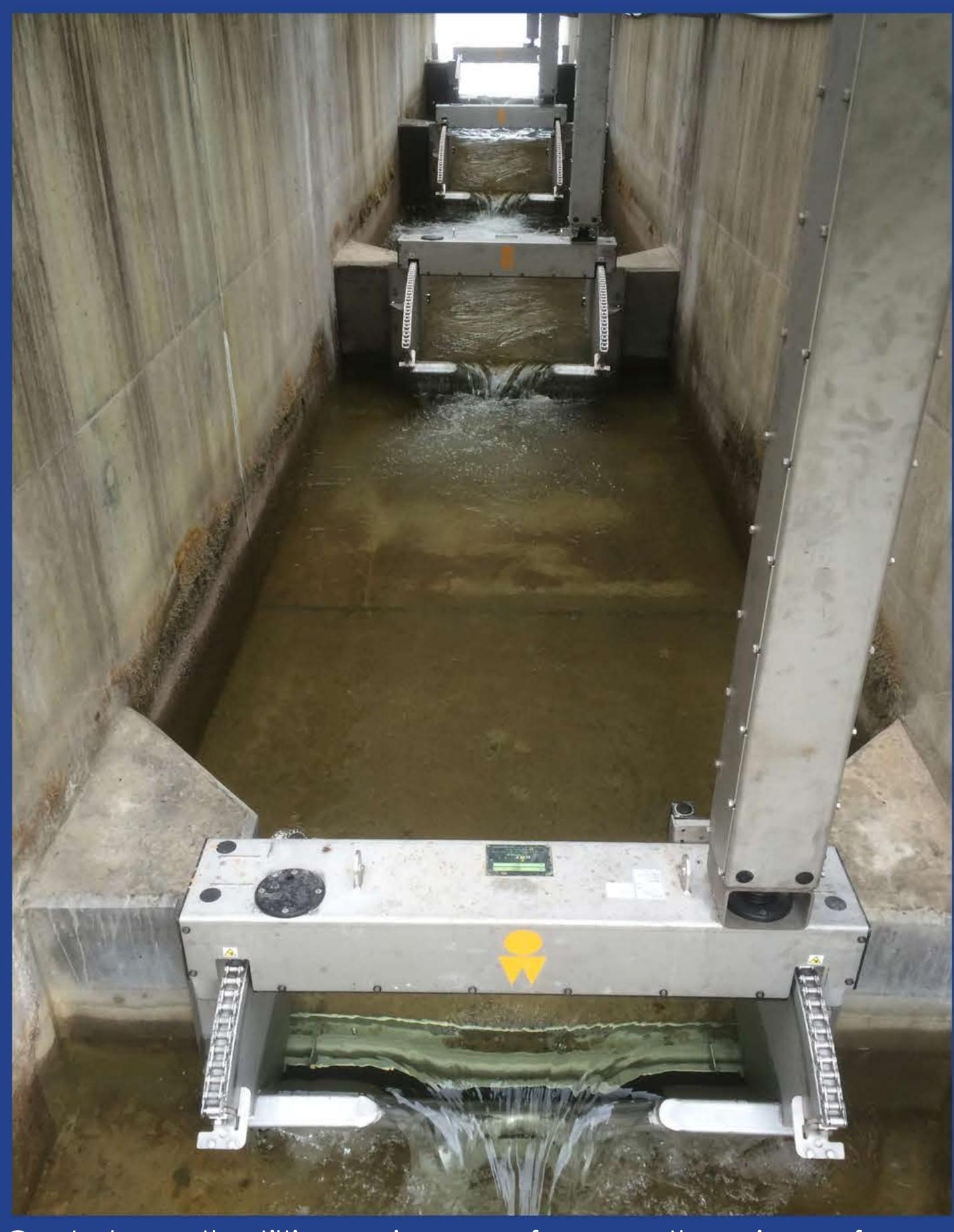
Control over the tilting weirs came from another piece of technology found in the water flow control industry. The "Greenbox" is a standalone unit, designed to sense water levels and adjust equipment such as a tilting weir to a suitable position. In the case of the fish pass at Loch Duntelchaig, this meant keeping the upper and lower water levels within the boundaries to allow fish passage.
