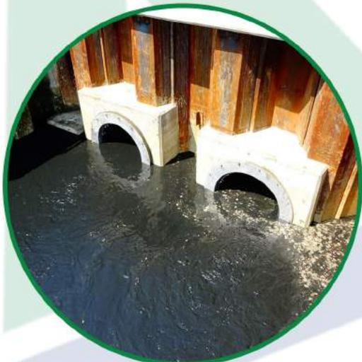
As part of the scheme, ACE worked closely with the Council to come up with the design of 2 new flood defences at Sterte & Creekmoor. By bridging the gap between the walls of 2 drainage channels, the new headwalls not only created a shortcut for pedestrians and cyclists, but also a home for the new WaStop valves. These allow water to drain into the harbour, but protect the channel from the high tides which were previously causing flooding.
