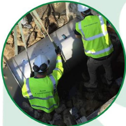
ACE supplied a number of WaStop valves in 2014. These covered a number of flood prone locations across the whole Harbour. Following the success of the previous project, ACE were asked to help with the design of further Flood Defences. Working with Avon Construction and Poole Council, ACE supplied 6 more WaStop valves. Ranging from 300mm diameter up to 1500mm. Two of which are the largest in the UK, to protect the area from tidal flooding.
