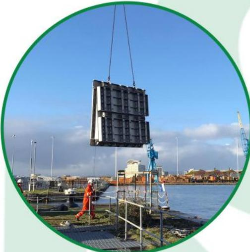
The ACE Technical team worked closely with the Sea-Lift Diving team to take into consideration the considerable difficulties the divers would face in fitting the flap valves. To ensure the fitting was as smooth and practical as possible minimal, chunky fittings were designed. This meant the divers could work quickly in the near zero visibility conditions faced 14 metres down. Once the design proposals and fitting procedures had been agreed the designs were sent to manufacture.
