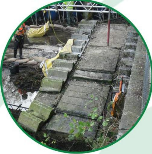
Thetford, a small market town in Suffolk, features an important crossing of the Little Ouse River and a large sluice gate structure which controls its levels, Thetford Sluice. The original sluice design lacked any fish pass facility but featured a canoe portage slope against the headwall. Inspections carried out by the Environment Agency (EA) and ACE concluded that a fish pass could be incorporated into the portage, whilst retaining its original use.
