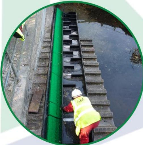
The simplicity of this product dramatically reduces the required amount of civil work needed, which reduces the cost of the overall project for the EA. In addition to the large cost saving of using HDPE in place of stainless steel, the ACE HDPE system significantly reduces the theft potential as HDPE has little or no scarp value. HDPE has a much lower material carbon footprint than a stainless-steel comparative.
